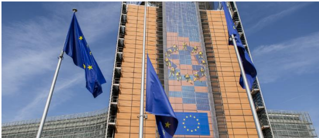
Berlaymont building, headquarter of the European Commission, Brussels, Belgium. Photo credits: Bogdan Hoyaux / European Union
